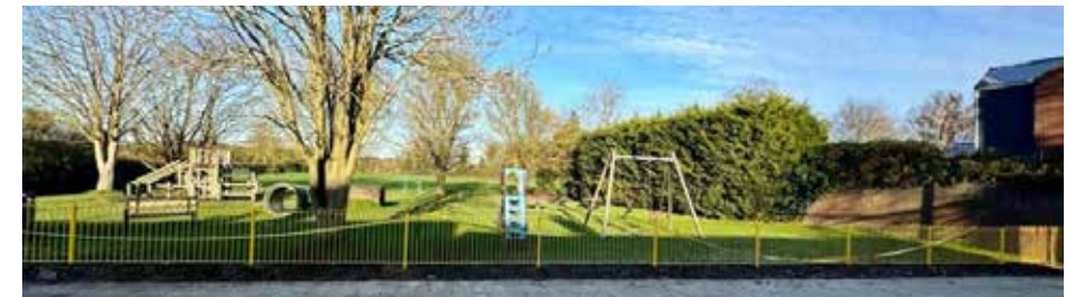
Chequer Street – Hedges removed, and new Fencing being installed.
